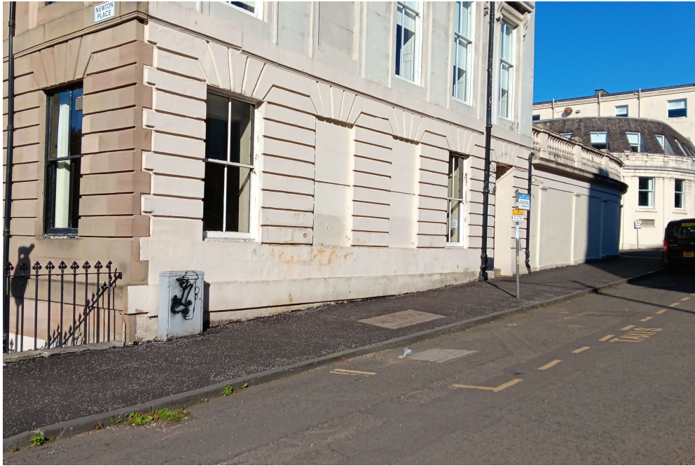
view of the building from outside
